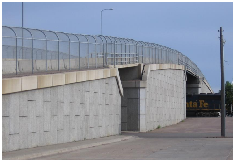
The Second Street Bridge provides a grade-separated vehicle, bicycle, and pedestrian crossing of the BNSF Railroad between the north side of the community and Downtown Aberdeen
