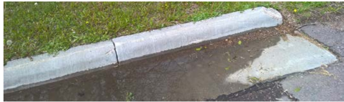
Curb with the rating of good.
