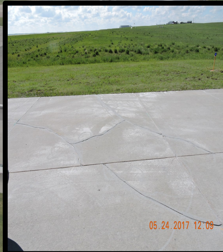
Saw and Seal Cracks
