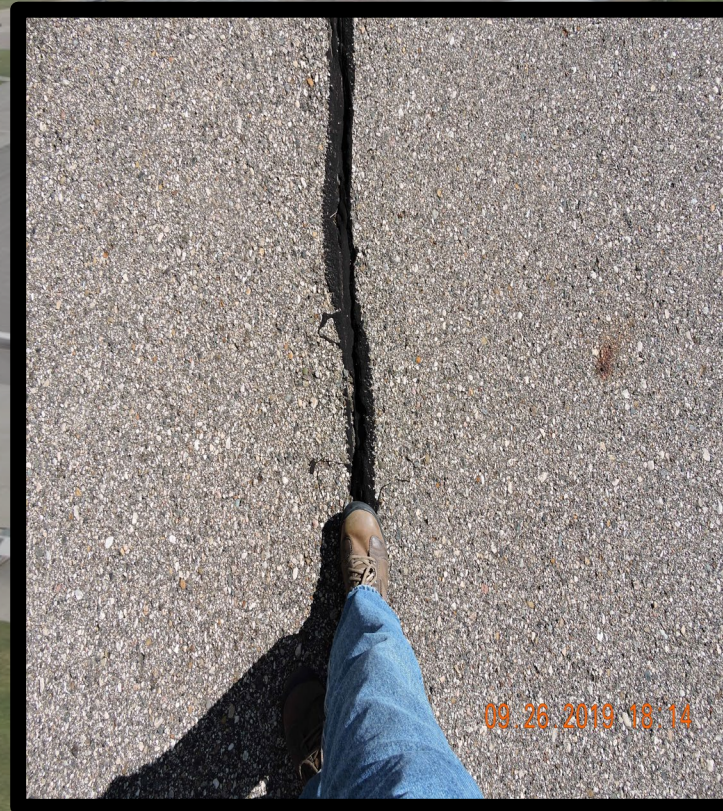
Crack Leveling
