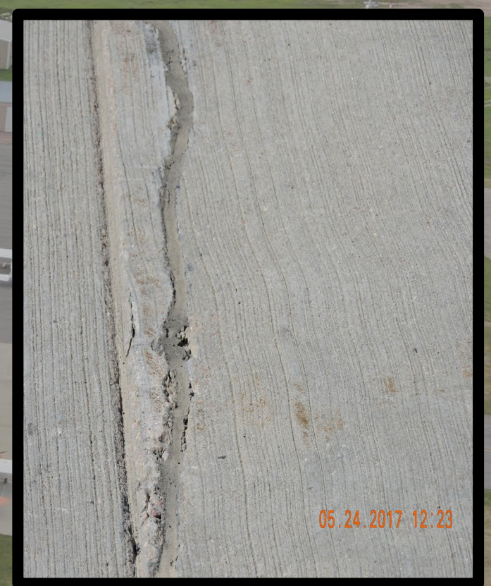
Corner Cracking
