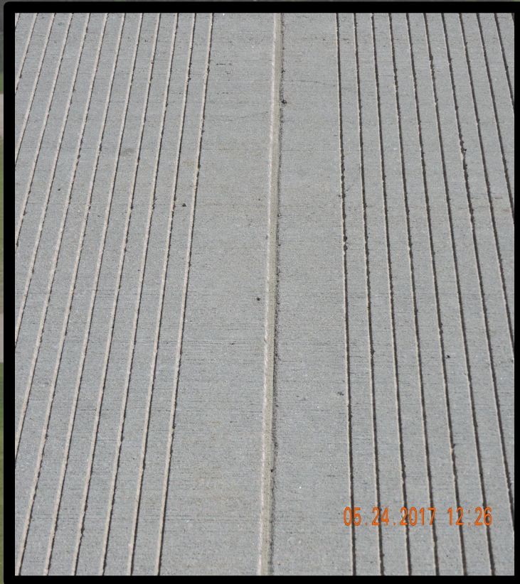
Saw and Seal Joints
