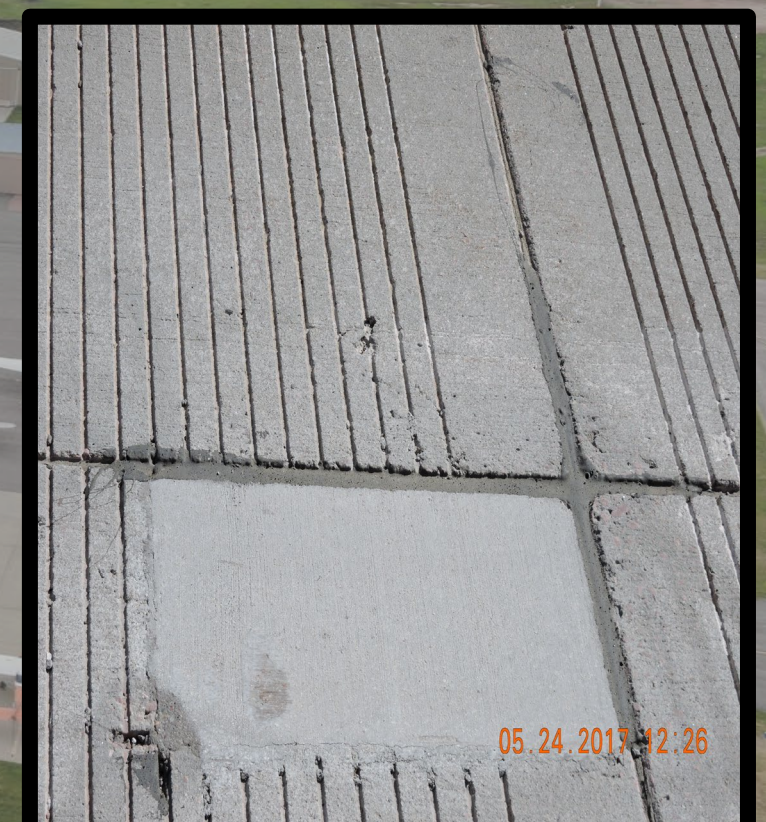
Spall and Corner Repair
