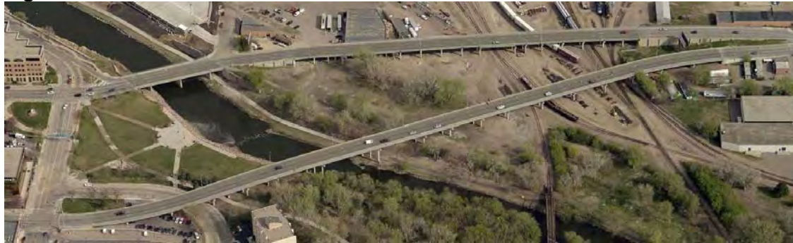
Figure 19.7 11th Street Viaduct
