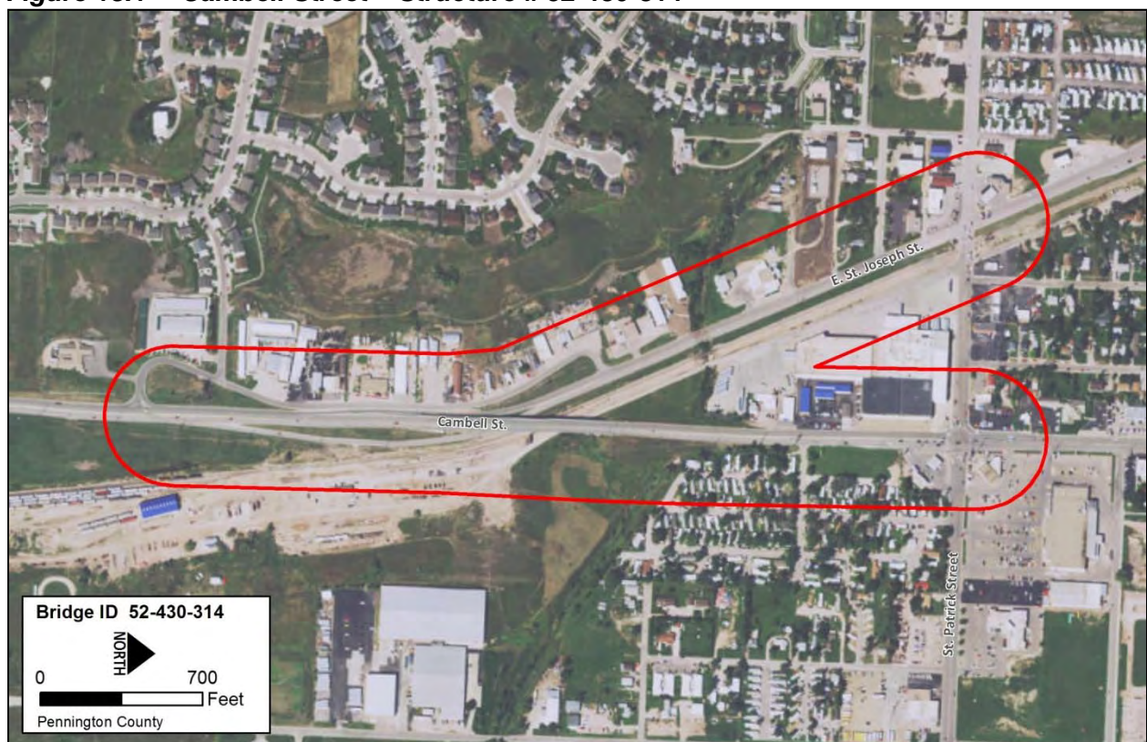
Figure 18.1 Cambell Street – Structure # 52-430-314
