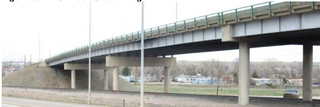
Figure 19.21 Cambell Street Bridge
