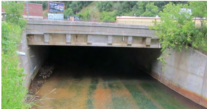
Figure 19.18 Deadwood Structure Outlet
