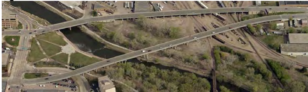
Figure 19.8 10th Street Viaduct
