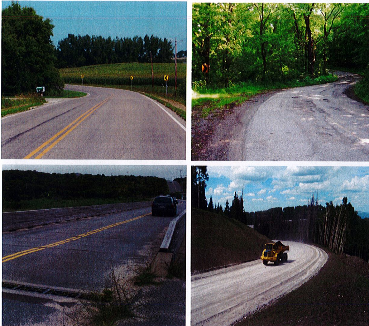
Figure 2-1. Typical Rural Low-Volume Roads (Source: CH2M Hill/Jacobs Engineering)
