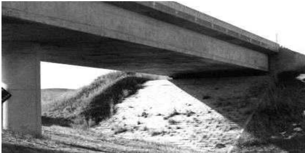
Figure 1.7 Concrete Rigid frame
