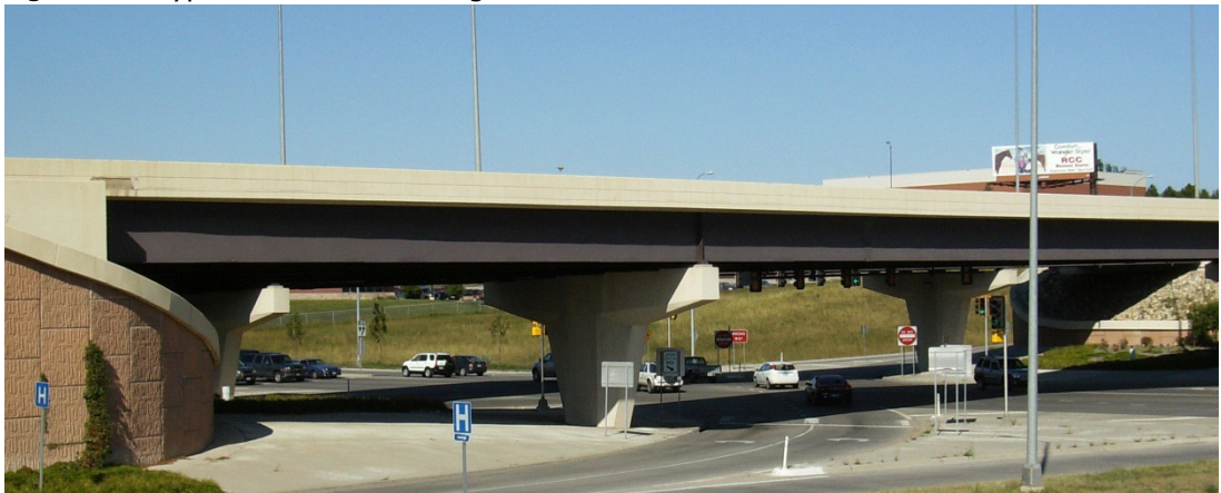
Figure 1.2 Typical Steel Girder Bridges
