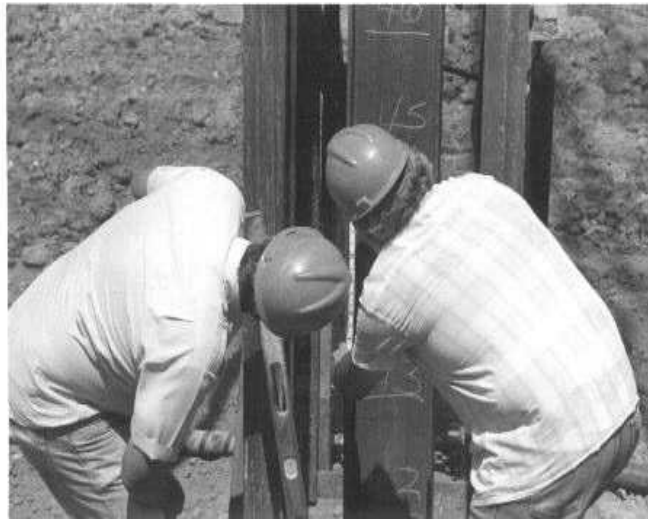
Figure 5.33 Driving a Steel Pile
