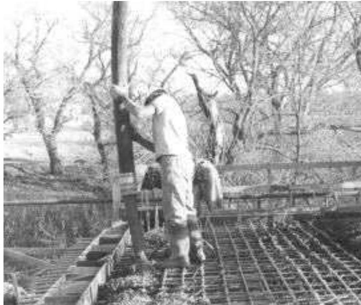
Figure 8.17 Discharge End of Pump Line
