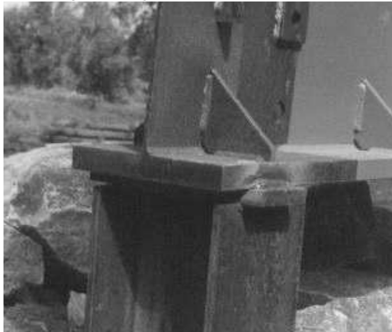
Figure 10.16 Bottom Flange to Bearing Plate Welds
