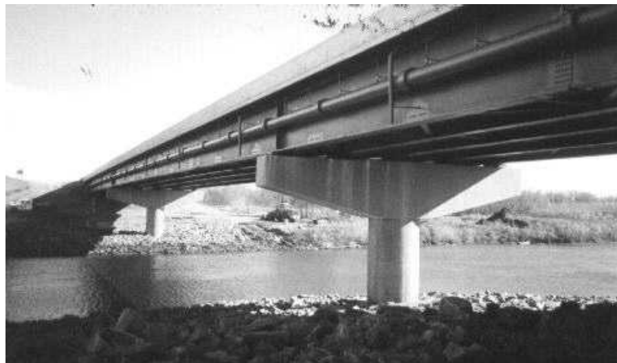
Figure 1.16 Typical Hammerhead Pier
