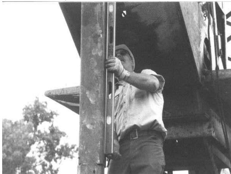
Figure 4.3 Plumb Check of Kelly Bar
