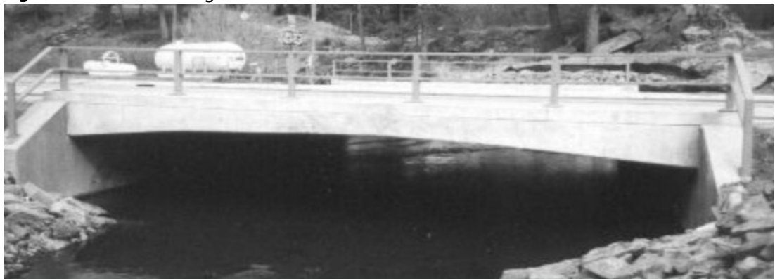
Figure 1.7 Concrete Rigid frame
