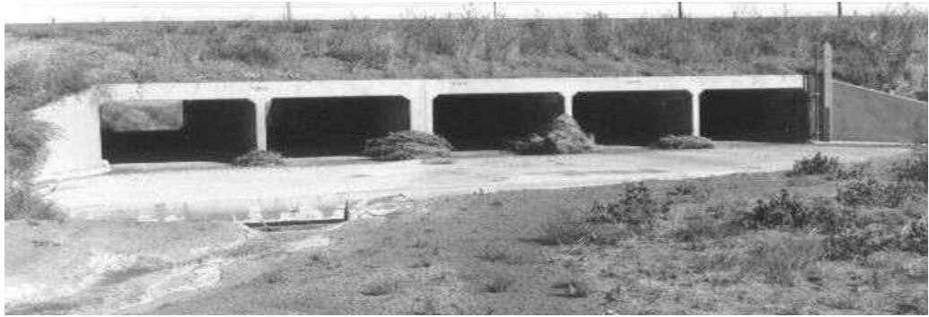
Figure 1.13 Typical Cast-in-Place Box Culvert
