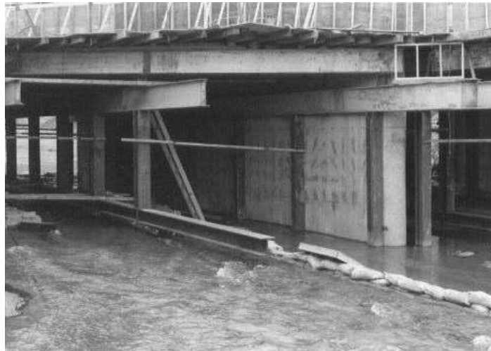
Figure 6.1 Typical Slab Bridge Falsework
