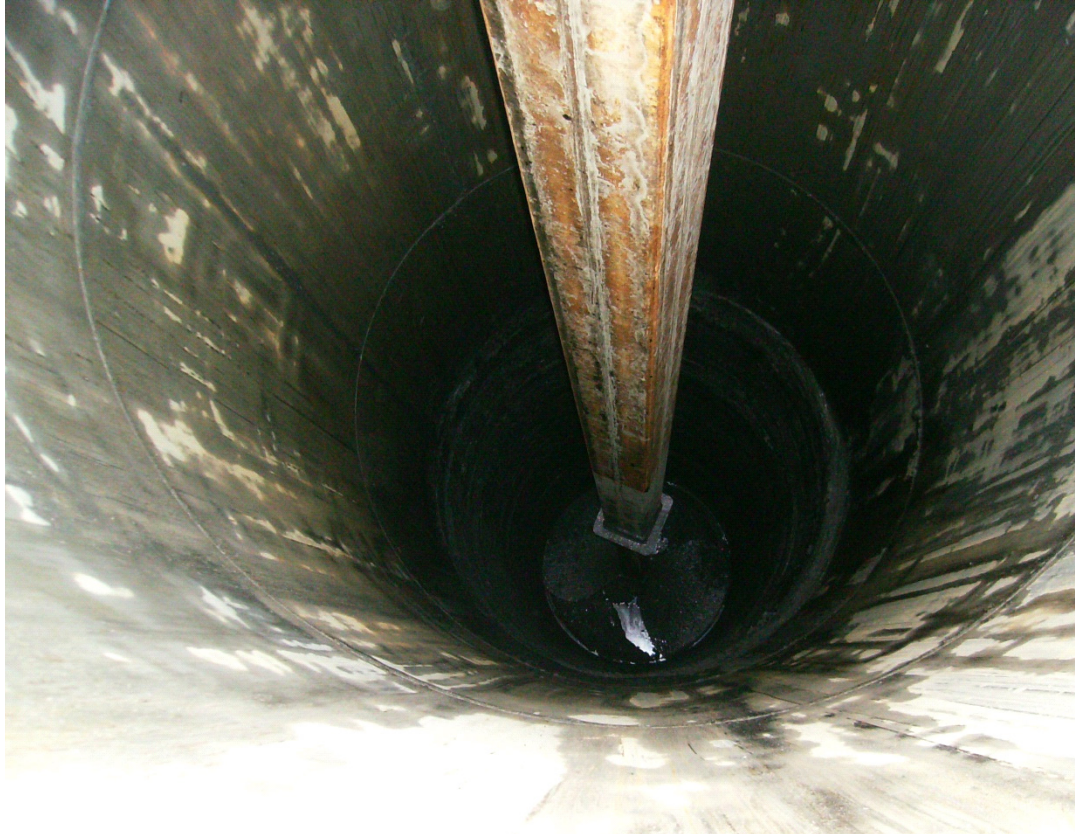
Figure 4.5 Drilled Shaft Casing
