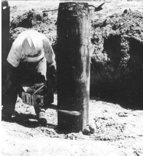
Figure 5.36 Cutting Off Timber Pile
