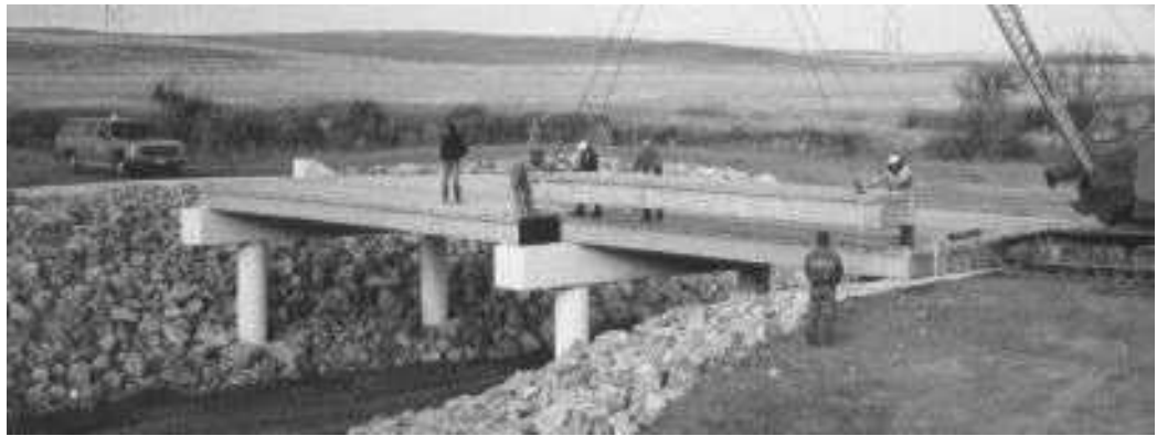
Figure 1.10 Bulb Tee Bridge
