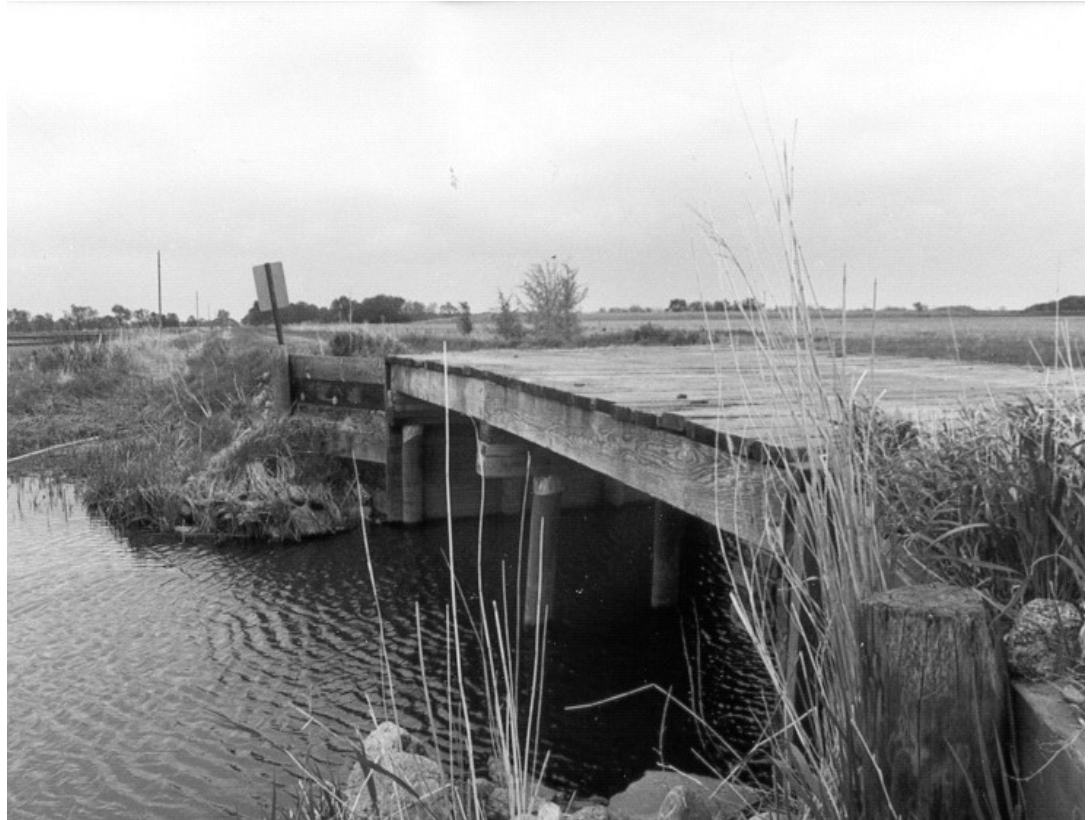
Figure 15.3 Typical Existing Timber Bridge
