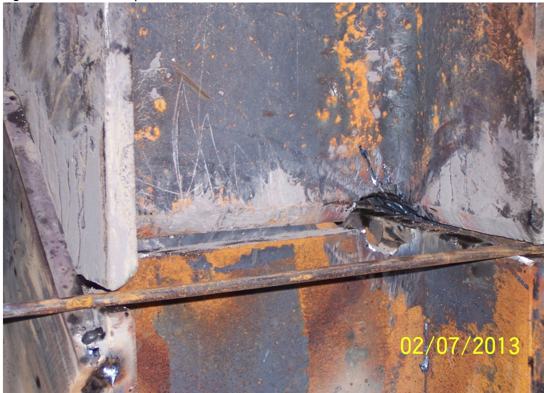
Figure 5.34 Steel Pile Splice
