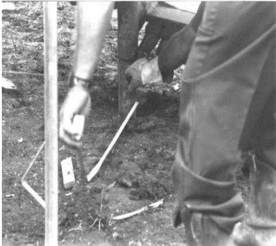
Figure 4.4 Measuring from Offset to Kelly Bar
