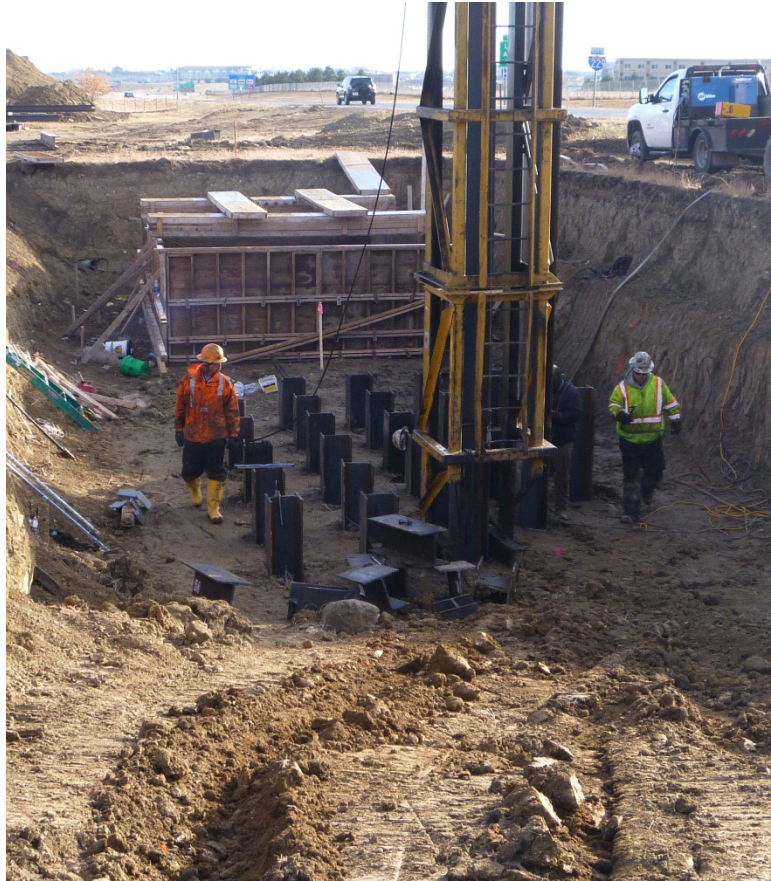
Figure 5.25 Driving Pile
