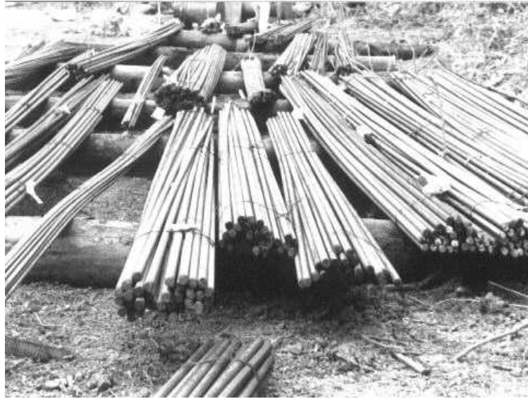
Figure 7.2 Reinforcing Steel Storage on Site
