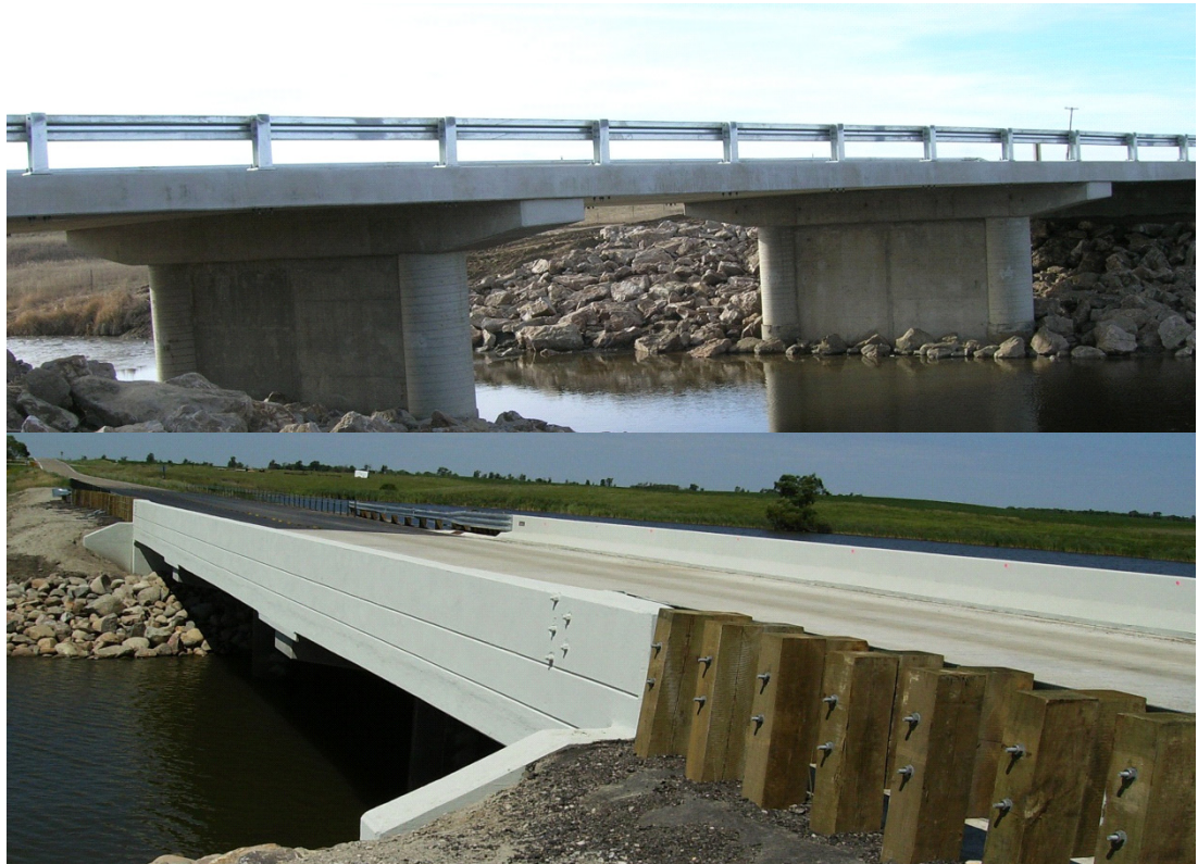
Figure 1.1 Typical Concrete Slab Bridges
