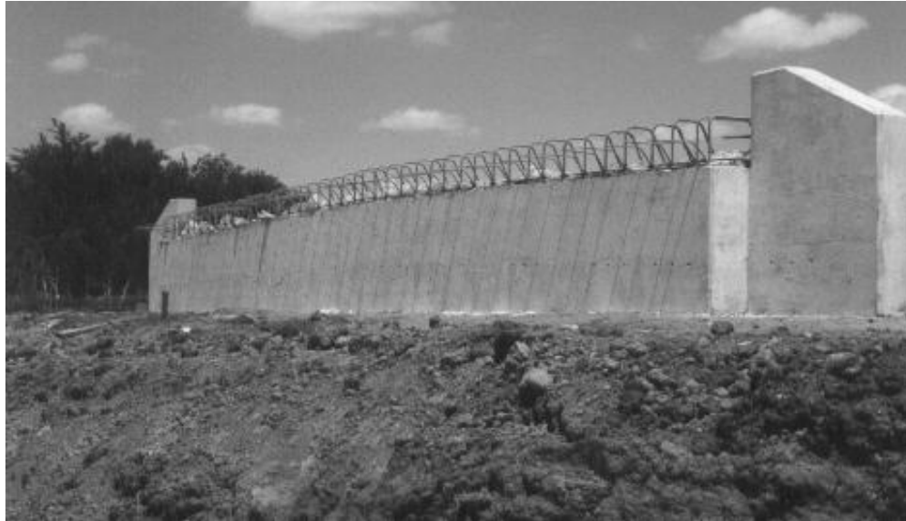
Figure 1.15 Typical Bridge Abutment and Wing wall
