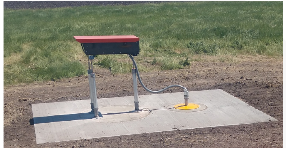
PAPI Installed on Concrete Foundation
