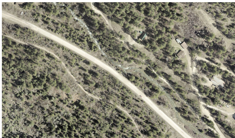
Aerial view of MRM 24 – Shoulder Widening Area
