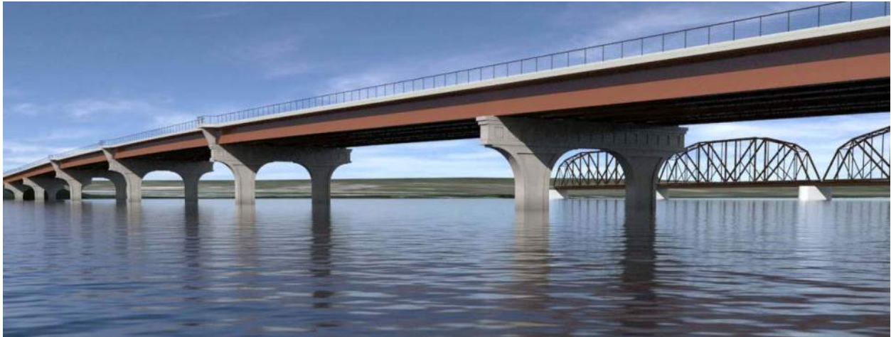
(a) Parallel Flange Steel Girder
