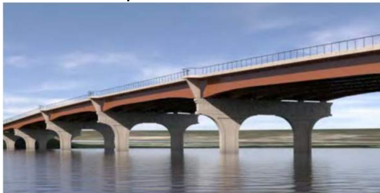
Figure 5.27: Steel Superstructure with Preferred Substructure
