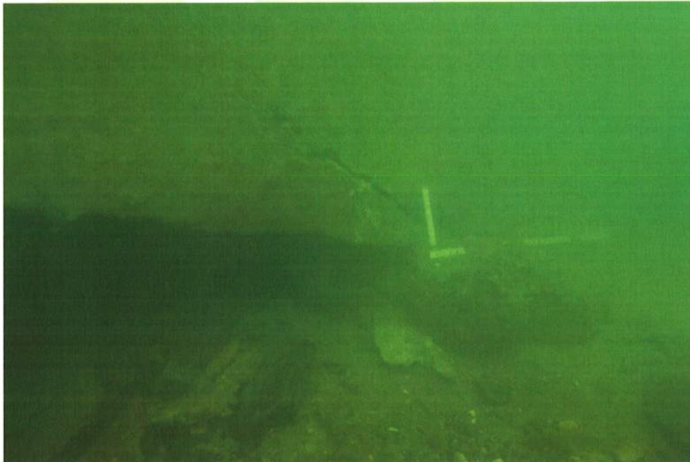
Photo 8 - Pier 6, Bottom of Footing, West Face
