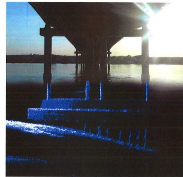
EAST ELEVATION ACOUSTIC IMAGE
