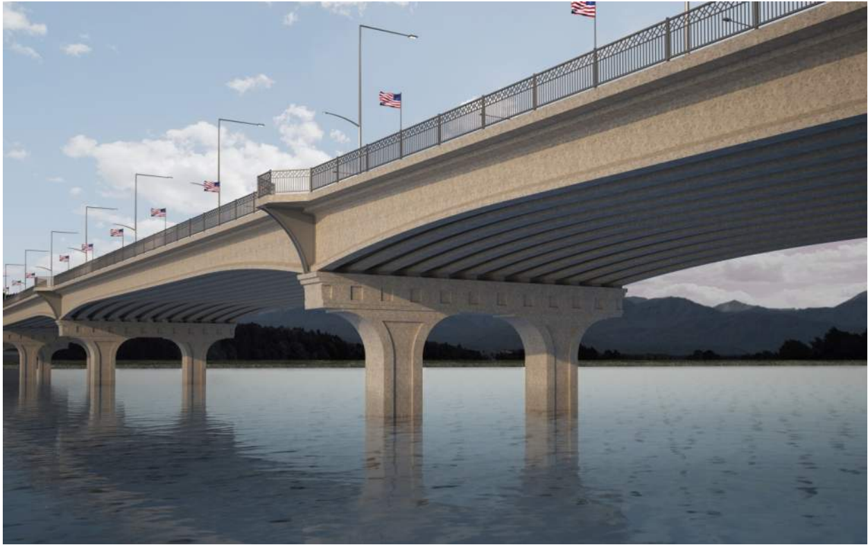
(c) Haunched Flange Concrete Girder
