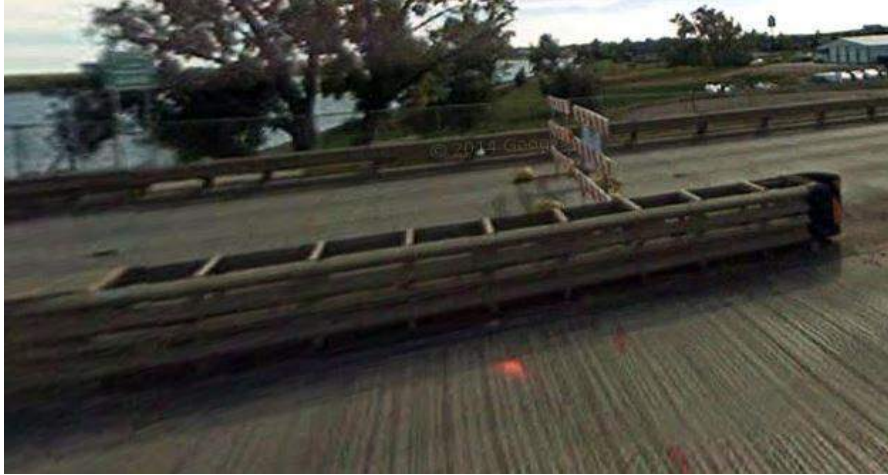
Figure 5: Crash Cushion at Western End of US 14 Missouri River Bridge
