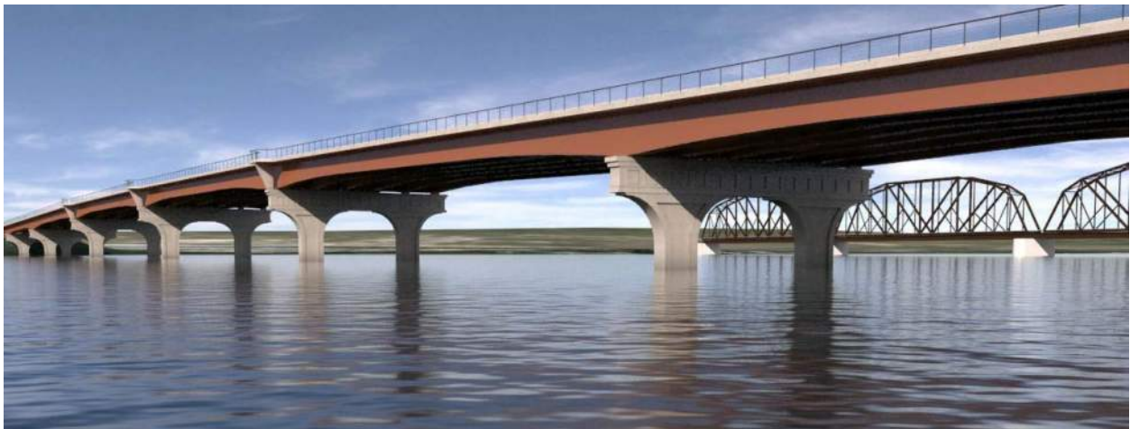
(b) Haunched Flange Steel Girder
