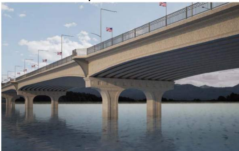
Figure 5.28: Concrete Superstructure with Preferred Substructure
