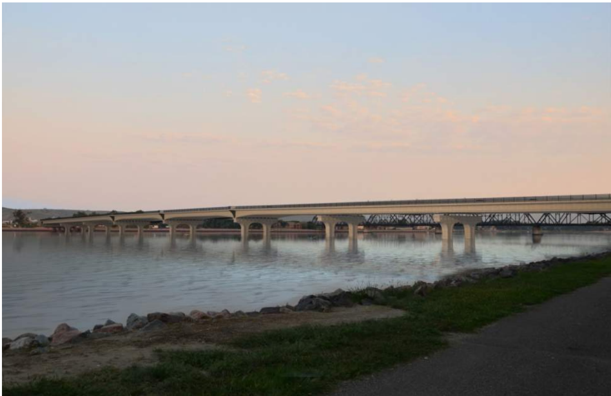
(d) Dual Column Pier with hybrid concrete beam layout – haunched mainspan, parallel approach
