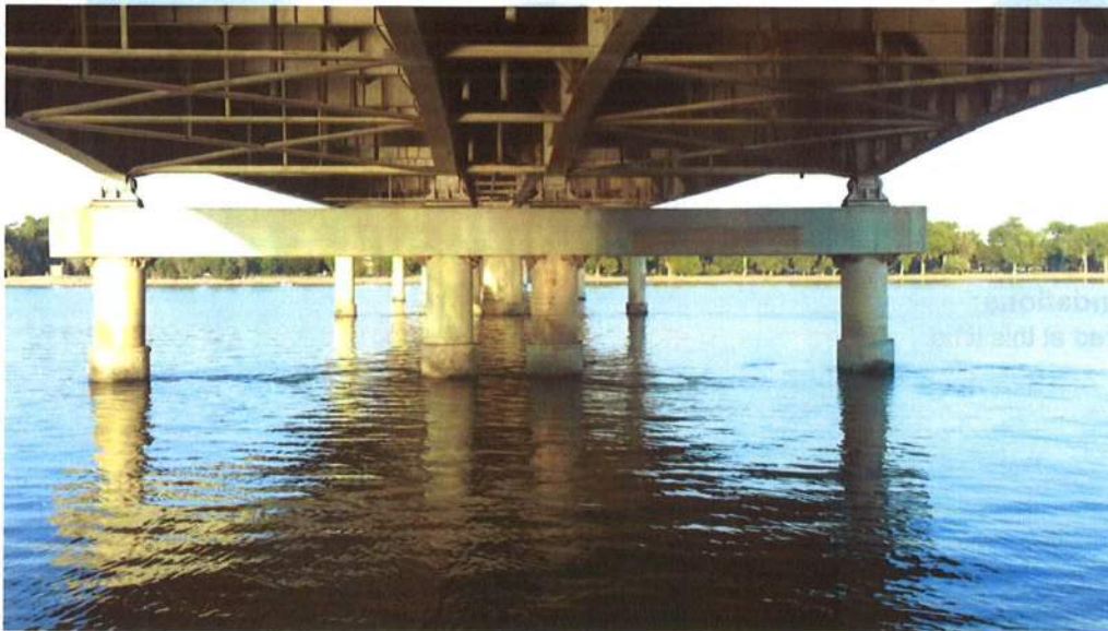
Photo 2 - Pier 3, West Face, Typical Substructure Configuration
