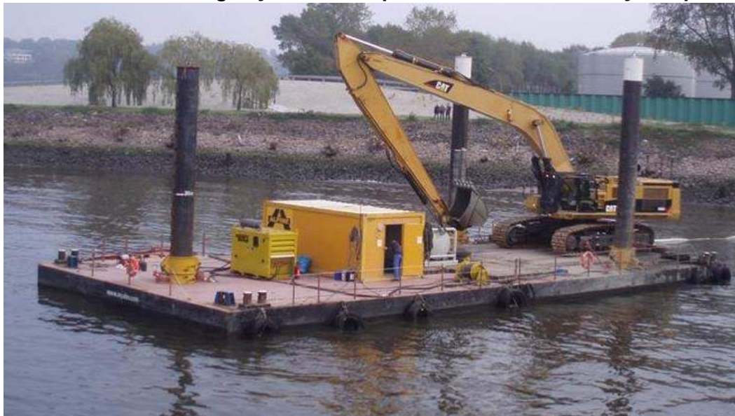
Figure 5:36: Modular Barge System with Spud Piles (Photo Courtesy of mpsbv.com)
