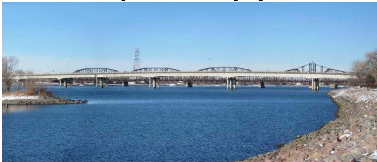
Figure 1.1 View of Existing Bridge
