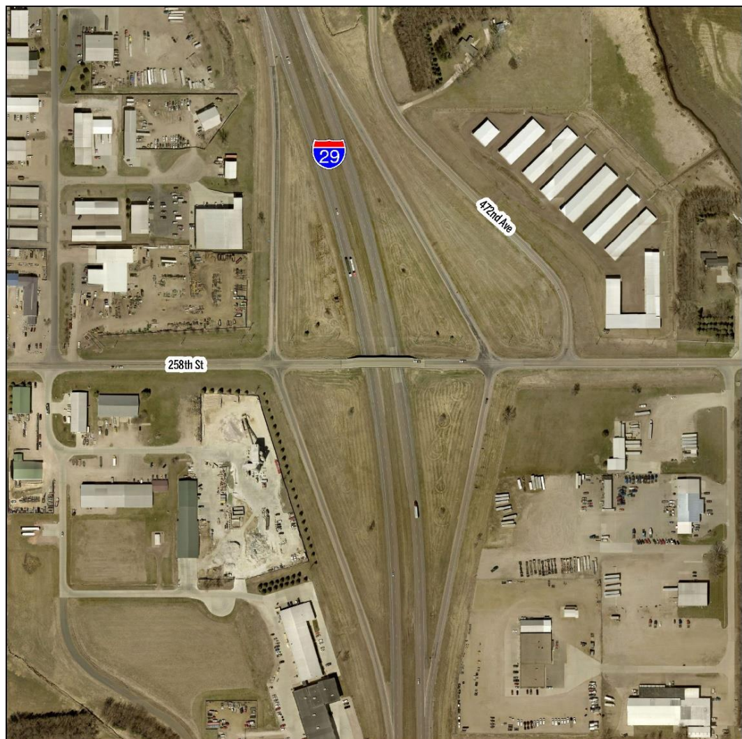
Figure 5 – Existing I-29 Exit 86 Service Interchange
