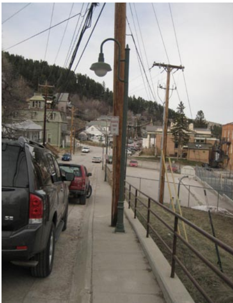
Williams Street is an example of efforts to provide sidewalks despite difficult construction conditions.
