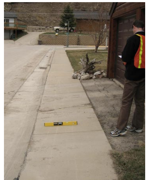
A field inventory of sidewalks included sidewalk termini, width, curb height, cross-slope, surface material, horizontal and vertical cracks, in-sidewalk obstructions, and curb ramps.
