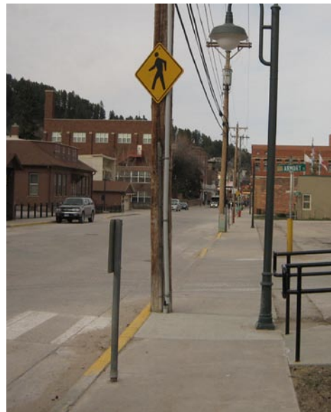
Crosswalks are well-signed, though a few locations should be brought into MUTCD compliance. An example is at the intersection of Upper Main Street and Armory Street where a downward arrow plate (W16-7p) should be installed.
