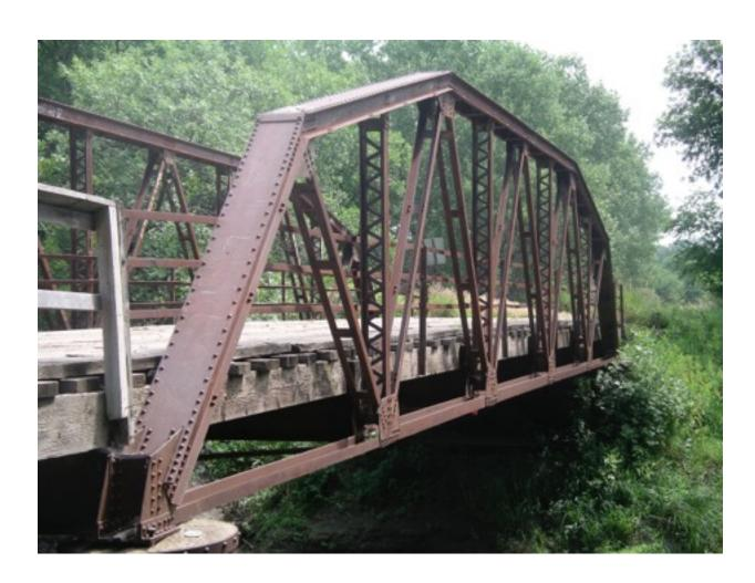
This riveted "Camelback" truss design is representative of truss bridges built in South Dakota after the 1910s.
