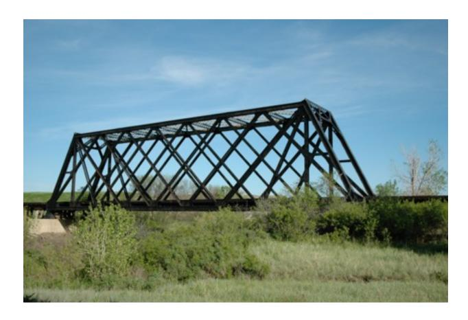
A multiple-intersection through truss bridges on the former Chicago & North Western line between Pierre and Rapid City -- one of the state's most distinctive bridge forms.
