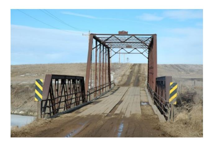
An example of an early pin-connected Pratt through truss bridge, with builders plates centered above the portals. The smaller span in the foreground is a Warren pony truss, of newer design.
