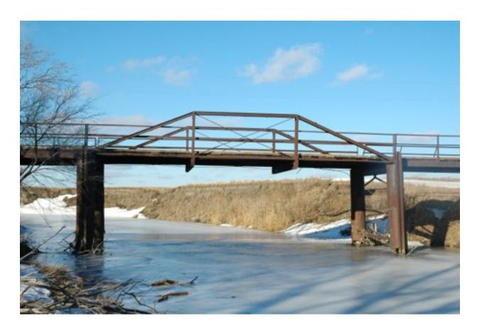
A small pin-connected Pratt pony truss bridge from the early twentieth century, with historic steel-caisson piers and steel stringer approaches. the 19th century, though they became a common bridge form in the early 20th.
