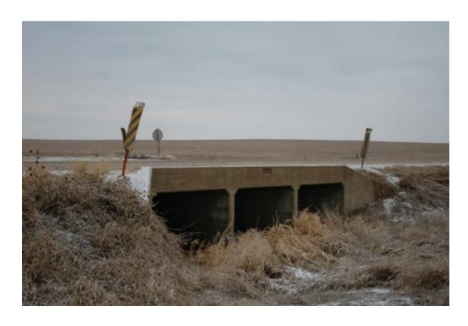
A typical three-barrel concrete box culvert from the 1930s.
