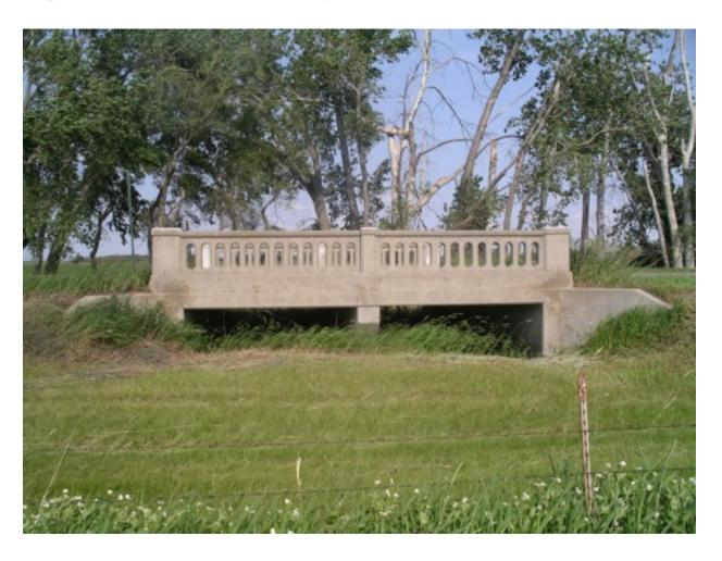
Most of the state's early concrete bridges featured a concrete balustrade with oval cutouts, rather than the pipe railings often used in later structures.
