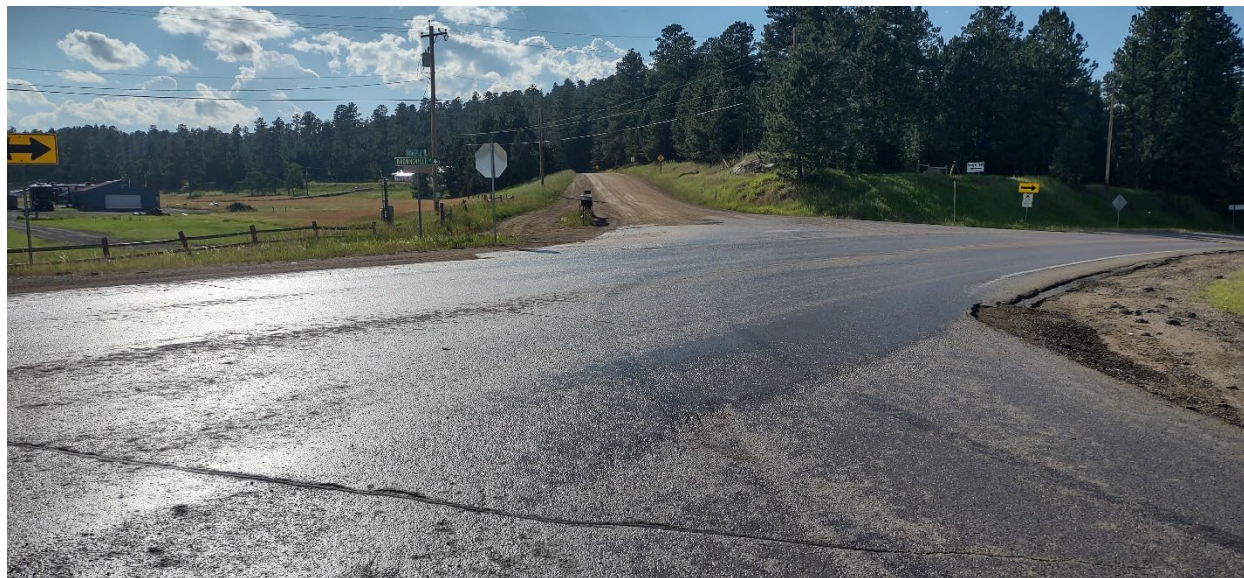
Figure 58. Study Intersection 15: Nemo Road and US Highway 385
