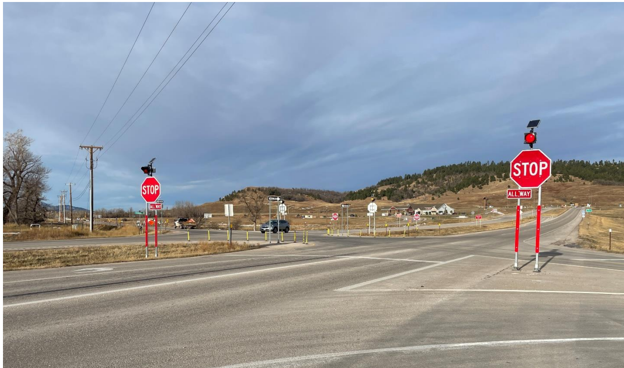
US85 & E. Colorado Boulevard/St. Onge Road Intersection (looking northwest)
