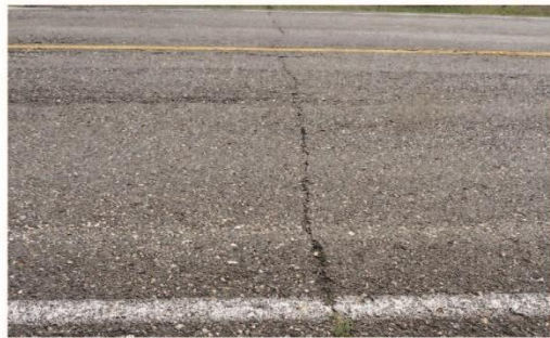
HIGH SEVERITY - Patch shows a high severity distress and/ or distinct roughness (greater than 25% of the section is affected)
