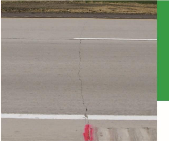
Low - Hairline to 1/4-inch wide cracks extending the full width of a panel.
