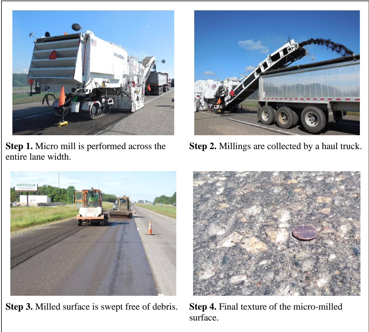
Figure 8. Micro-Milling General Construction Steps.
