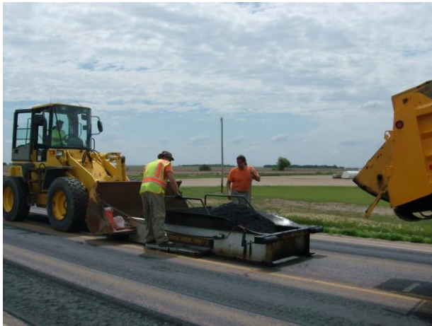
Step 3. Placing mix with Yankton box.
