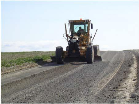
(a) Placing Gravel Surfacing
