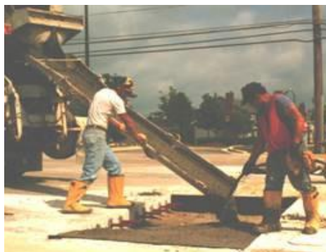
Step 5. Material placement. Conventional PCC material is most common for full-depth repairs.
