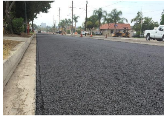
Step 4. Finish mat before rolling.
