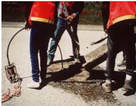
Step 7. Repair material placement. Material should be placed per governing specifications.
