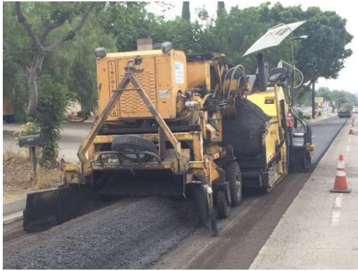
Step 3. Paving machine.
