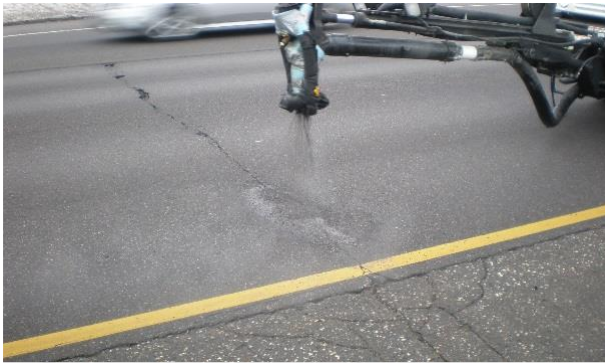
Step 3. The slurry is used to fill the pothole.
