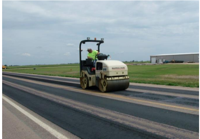
Step 6. Rut filling almost complete.
