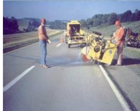
Step 2. Concrete removal. Sawing the boundaries and removing deteriorated PCC.
