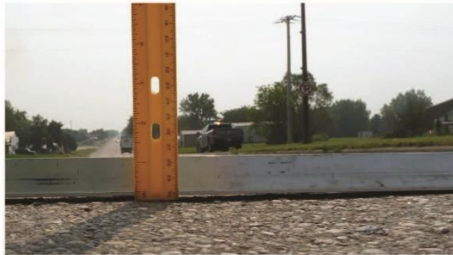
Low - Depressions in the wheel path less than 1/8 inch.
