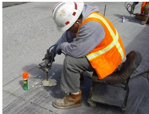
Step 4. Plug injection hole.
