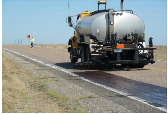
Step 2. Spraying tack coat.
