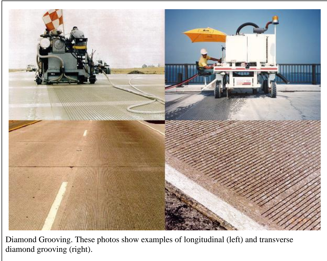
Figure 23. Diamond Grooving General Construction Steps.
