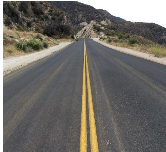
Step 6. Finish mat after flush coat.
