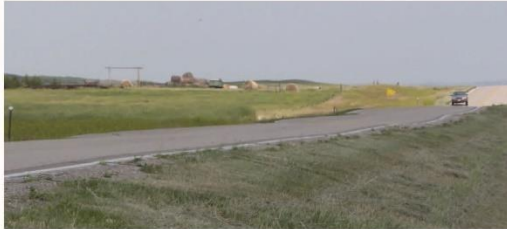
Low - Slight waves, sags, humps, corrugations or wash boarding of the pavement.
