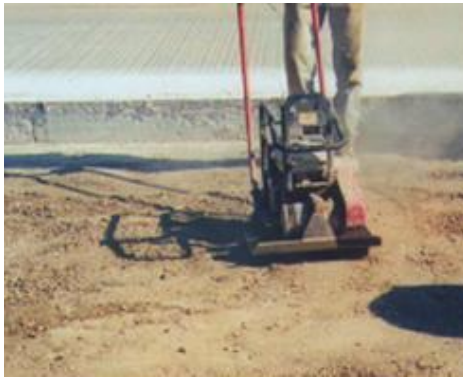
Step 3. Repair area preparation. It is important that the repair area be dry and properly compacted.
