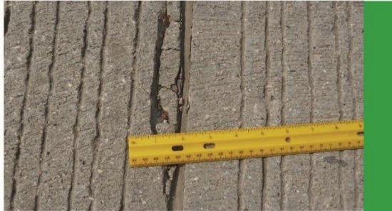
LOW SEVERITY - Spalls less than 3 inches wide with no significant loss of material or Joint & Spall Repair Patch with cracking (1% to 9% of the joints are affected)
