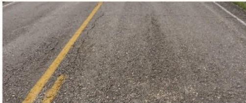
MEDIUM SEVERITY - Patch shows low or medium severity distress and/ or notable roughness (10% to 24% of the section is affected)
