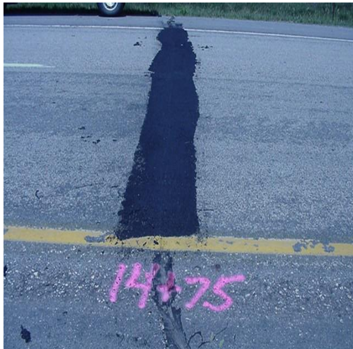
Step 2. Finished product after leveling.
