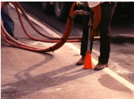
Step 3. Inject material beneath the slab.
