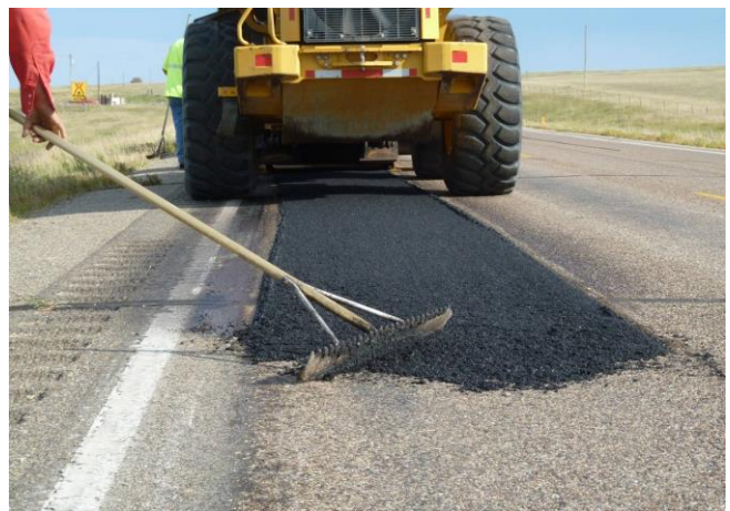
Step 4. Raking mix to create a smooth transition.
