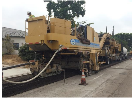
Step 2. Milling machine.
