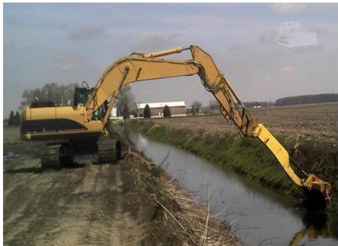
(b) Cleaning drainage ditch.
