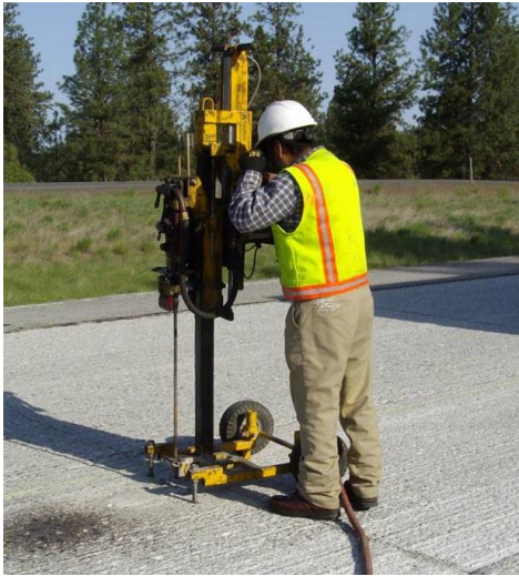
Step 1. Drilling of injection holes.
