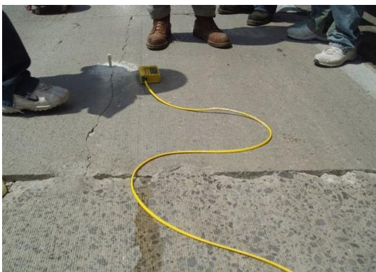
Step 5. Monitor the amount of lift using traffic.
