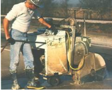
Step 1. Concrete sawing. Repair boundaries are cut with full-depth, diamond-bladed sawing.
