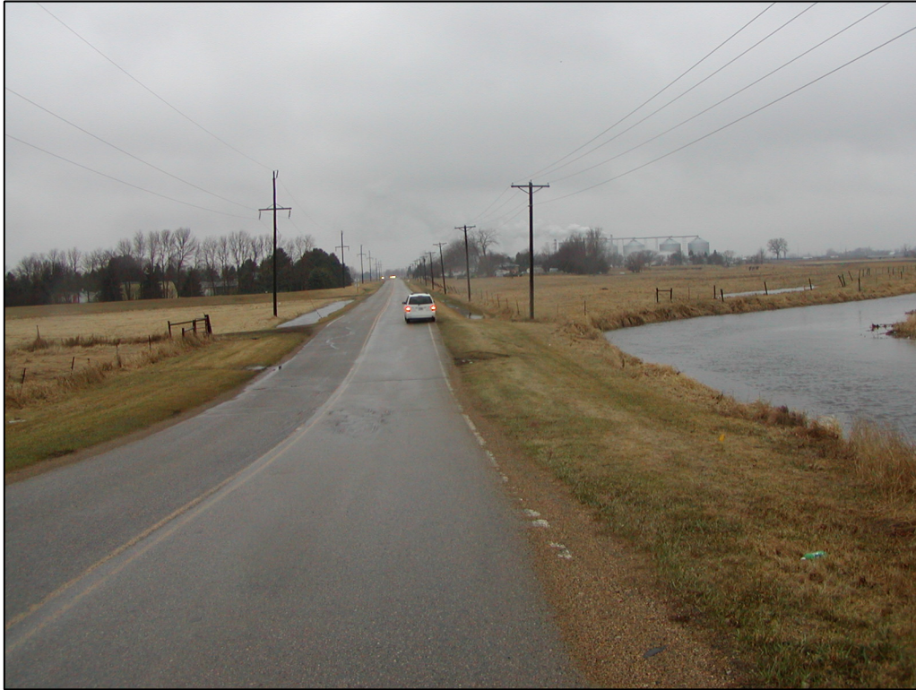
Photo 3 Looking west at spillway and away from bridge
