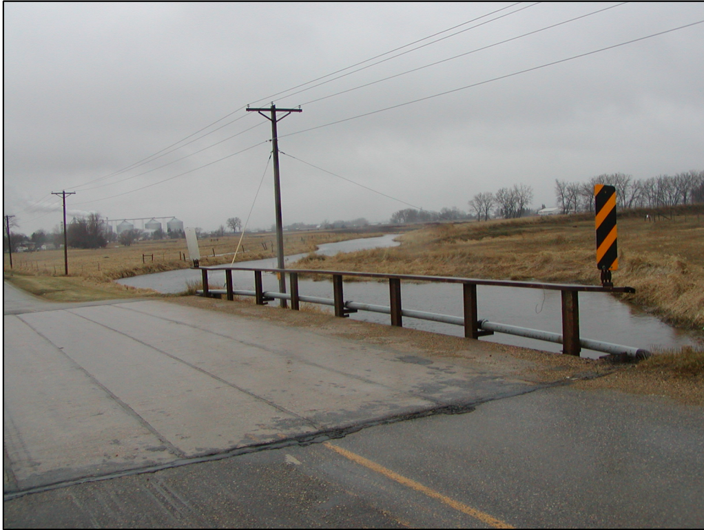
Photo 1 Looking northwest (upstream) from 20th Avenue South bridge
