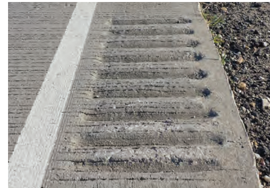
Rumble strip in portland cement concrete
