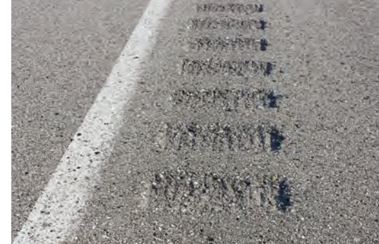
Rumble strip in asphalt concrete shoulder
