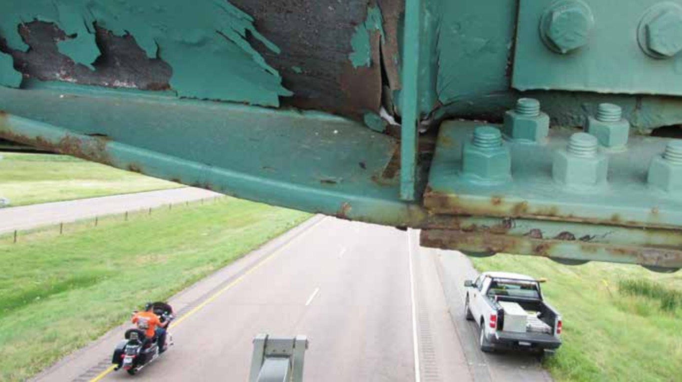
Above: A steel girder on the Hartford exit overpass damaged by an Aug. 2016 hit. Right: Damage to the same bridge in 2014. The total for heat-straightening steel girders and replacing other bridge parts for both hits was more than $1 million.
