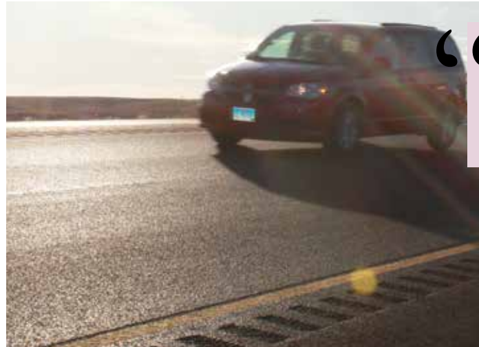
Rumble strips line both sides of the northbound and southbound lanes of U.S. Highway 83, a newly resurfaced divided highway in Stanley and Lyman counties.
