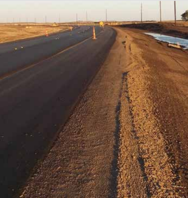
2018 shoulder-widening project in Perkins County
