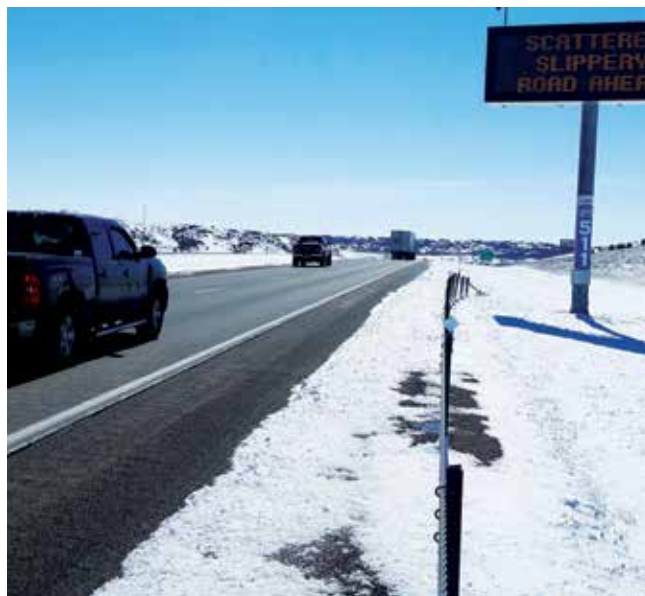
Dynamic message signs like this one near Oa-coma are part of SDDOT efforts to inform the traveling public of real-time road conditions.
