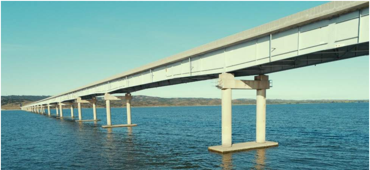
The Platte-Winner Bridge features a girder-style construction that is repeated across all spans.
