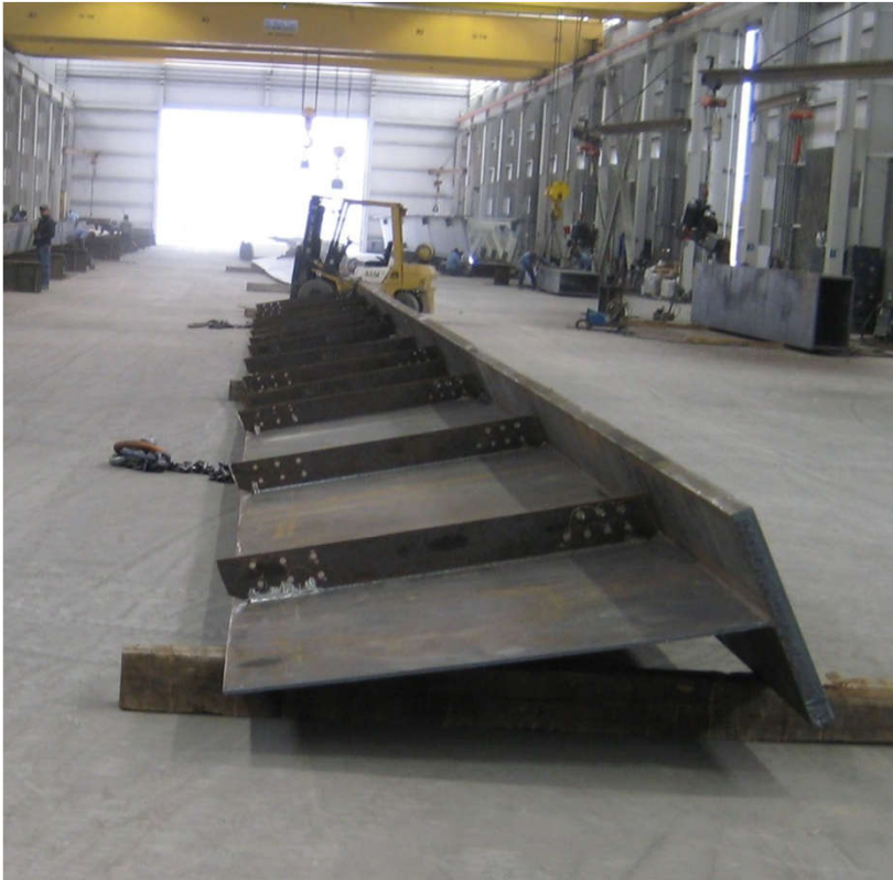
Flanges and Connection Plates Welded to Web
